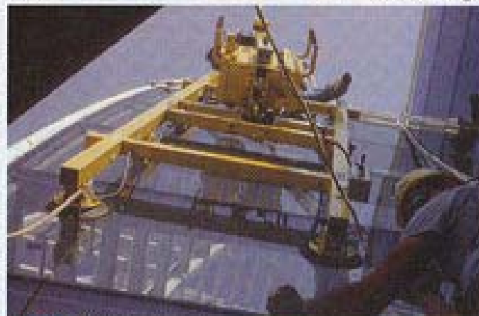
UNITIZED Skylight glass installed in preglazed units.
