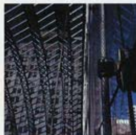
TRANSPARENCY Vaulted skylight meets glass end wall, called unique.
